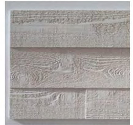
BOARD-FORMED CONCRETE PANEL TO REFERENCE HISTORIC CRIBBING
